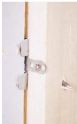
Figure 3. Drywall clips, installed about 12 inches apart, offer an alternative approach to floating corners and eliminate the need for the third corner stud or backup framing along ceiling edges.
