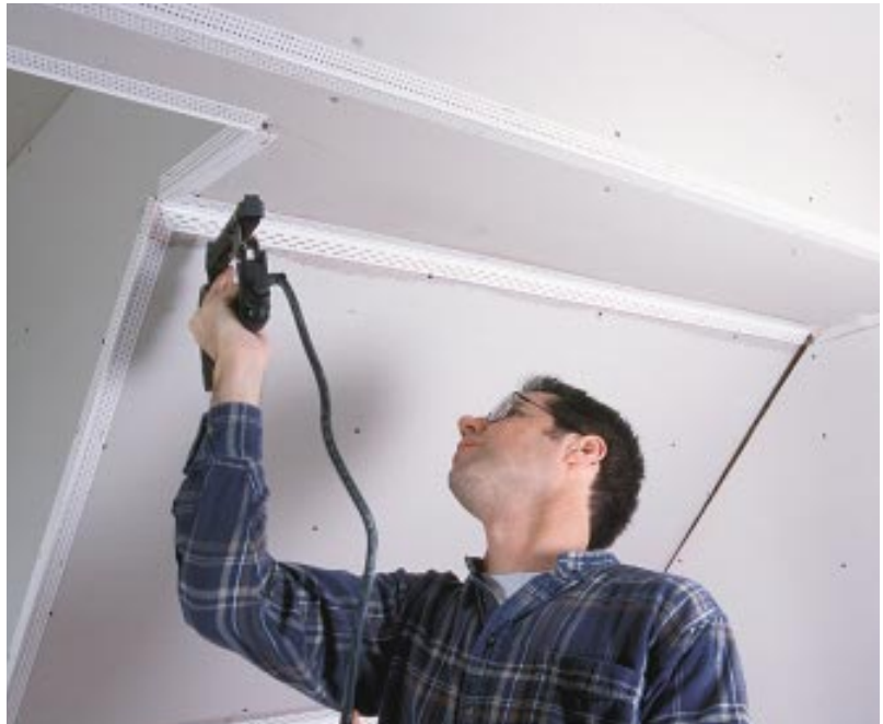
Figure 5. Mud- or glue-on perforated vinyl corner beads that move with the drywall, not with the framing, eliminate bead pops and make ding repairs a snap.
