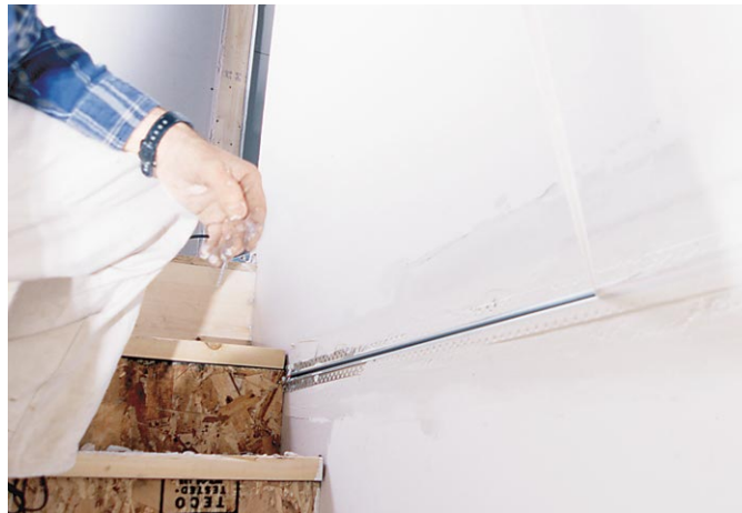
Figure 6. Expansion joints can prevent ridging at tall expanses of drywall, as in stairwells. The joint can be painted to blend in or be concealed by trim.
