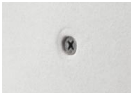
Figure 1. To minimize nail pops, keep the drywall tight to the framing and choose the right length fastener. Screws should penetrate the framing by \frac{5}{8} inch, nails by \frac{7}{8} inch. The screw or nail head should indent, but not break, the paper facing.
