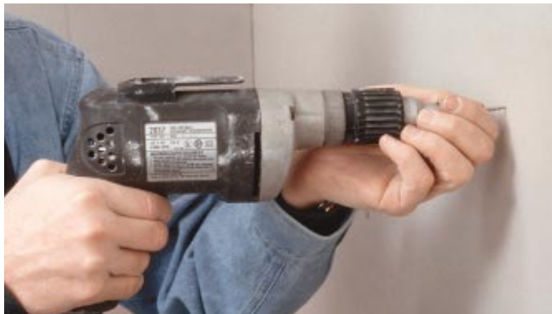
Figure 1. To minimize nail pops, keep the drywall tight to the framing and choose the right length fastener. Screws should penetrate the framing by \frac{5}{8} inch, nails by \frac{7}{8} inch. The screw or nail head should indent, but not break, the paper facing.
